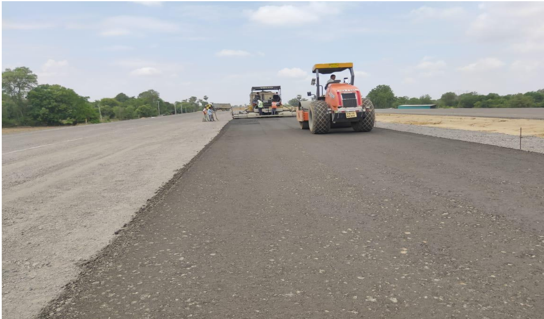
WMM laying in progress
