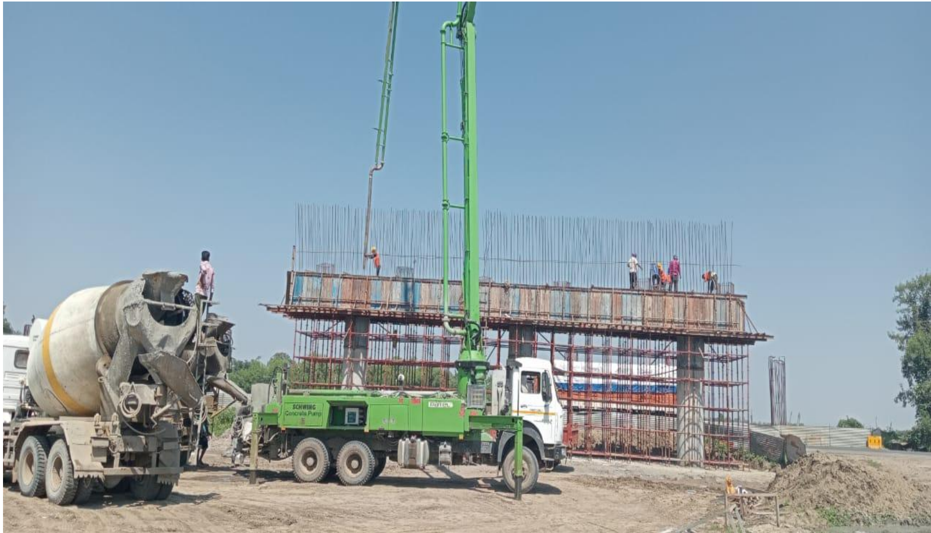
A 2 Pier cap casting at Ch. 364+746 VUP (LHS)
