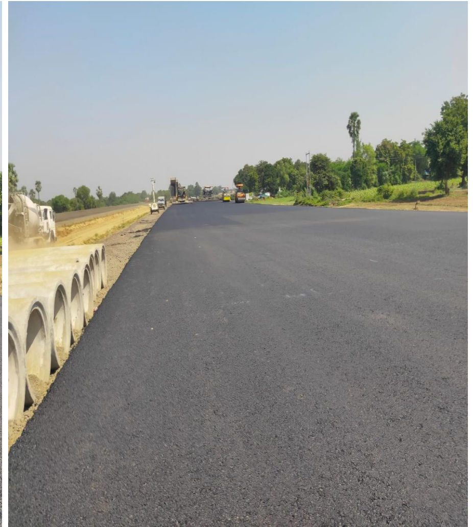
DBM 2nd layer laying at Ch. 356+390 to 356+760 (LHS)
