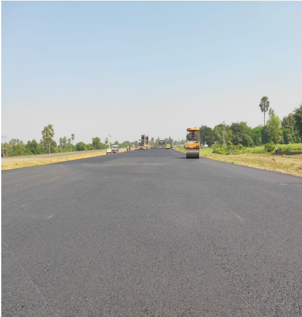
DBM 2nd layer laying at Ch. 356+390 to 356+760 (LHS)
