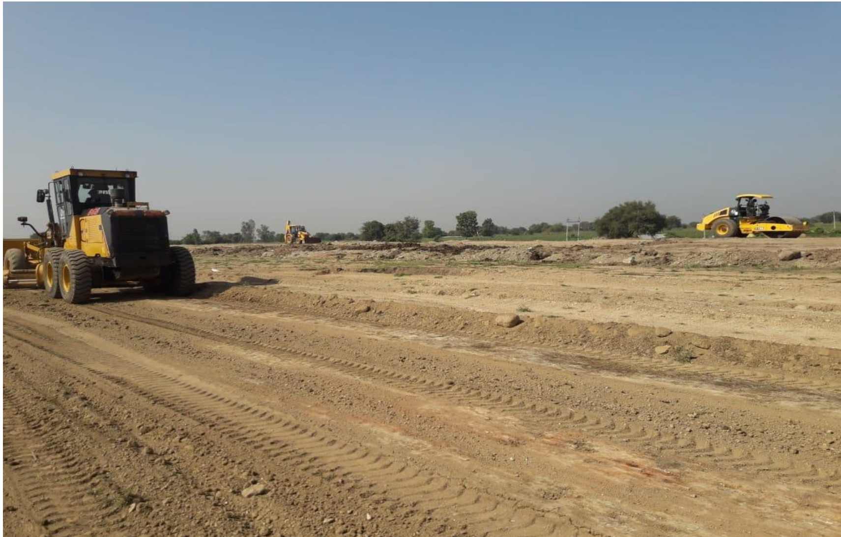
Embankment Layer in progress
