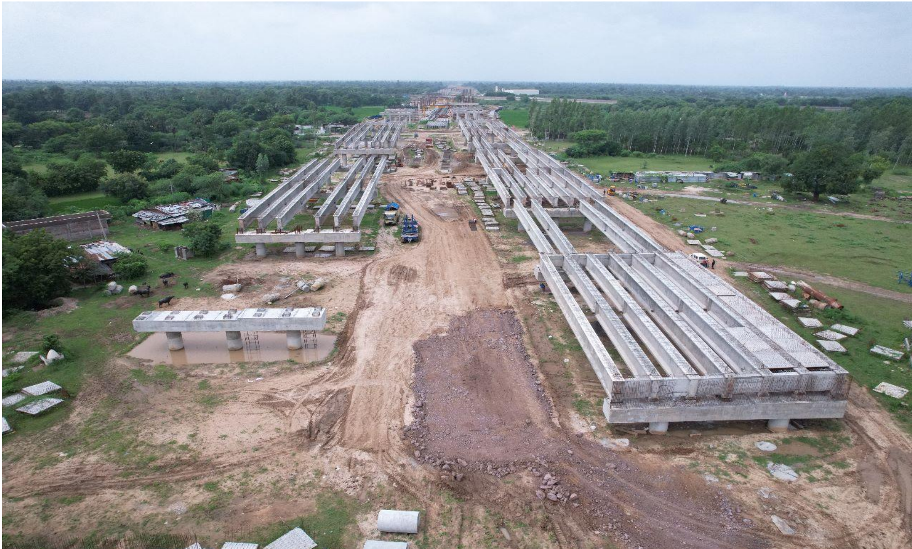
Work In Progress at Major Bridge ch. 352+281
